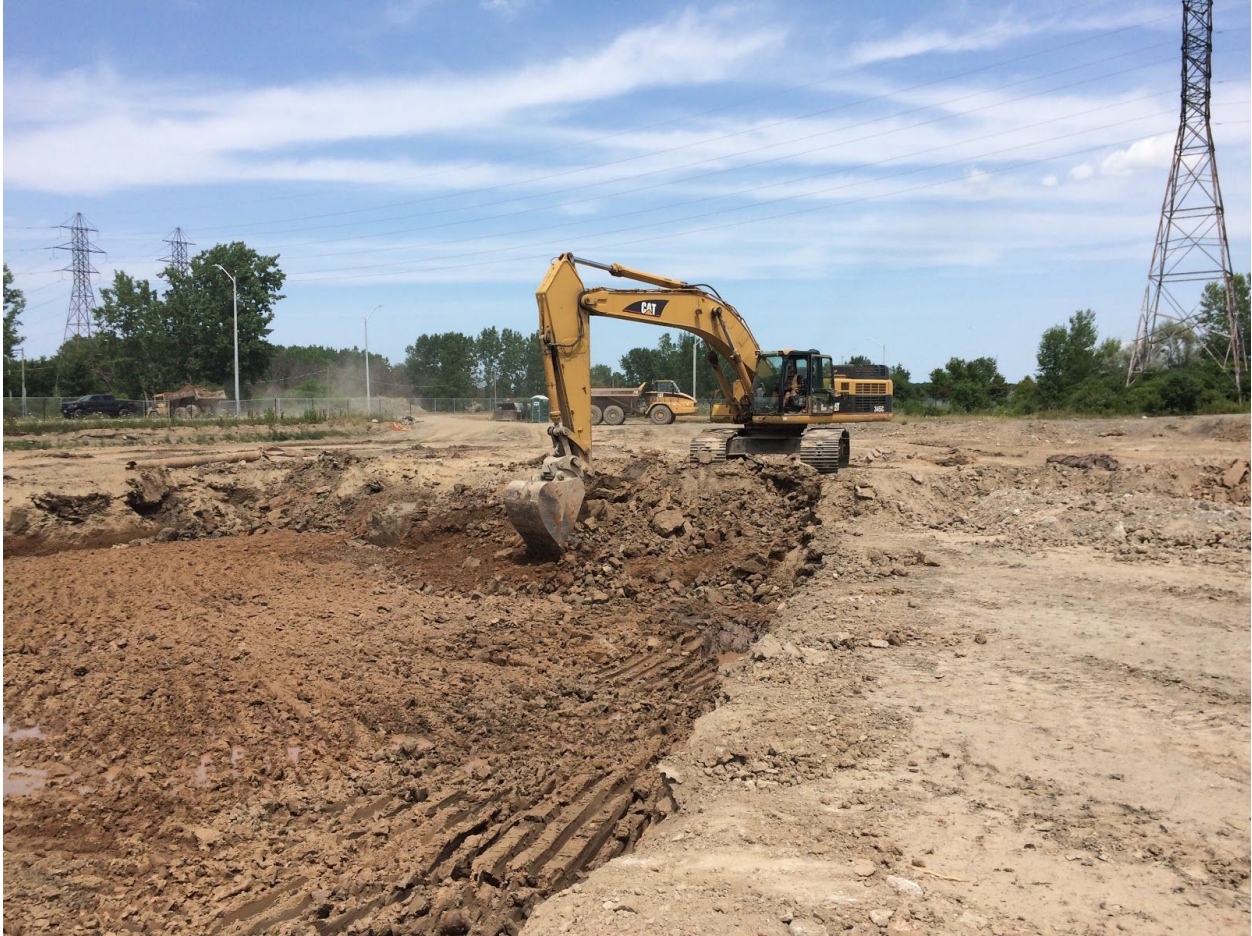
Figure 1; Excavation. (© 2019, 1939522 Ontario Limited, Tim Collins)
