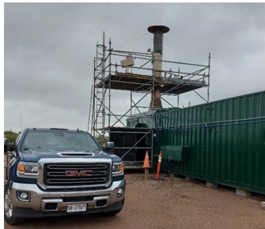
Dillon Testing Equipment in place/Stack created to conduct emission tests. August 2021
