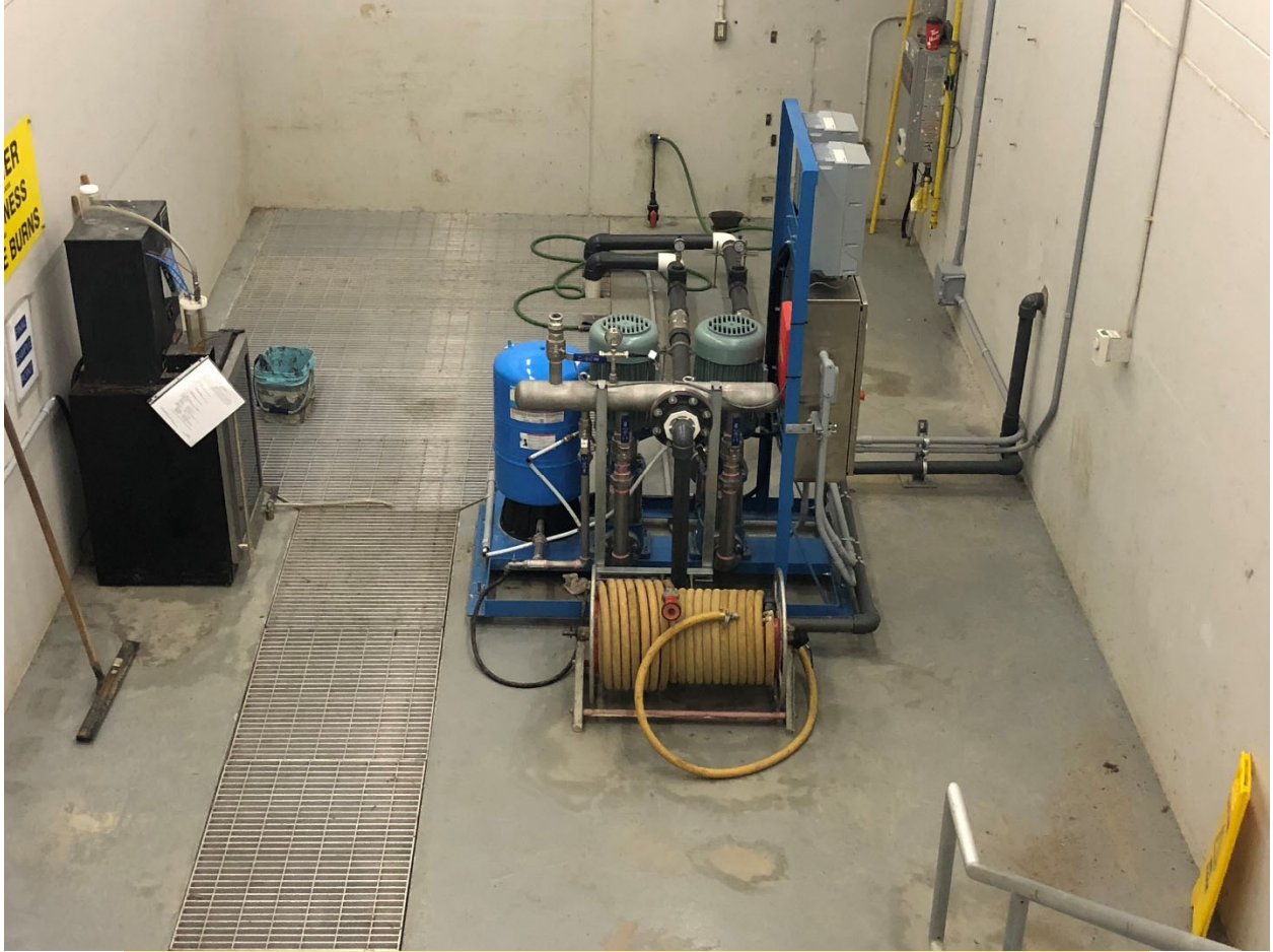
PICTURE OF EFFLUENT CHANNEL AFTER INSTALLATION OF REUSE SKID
