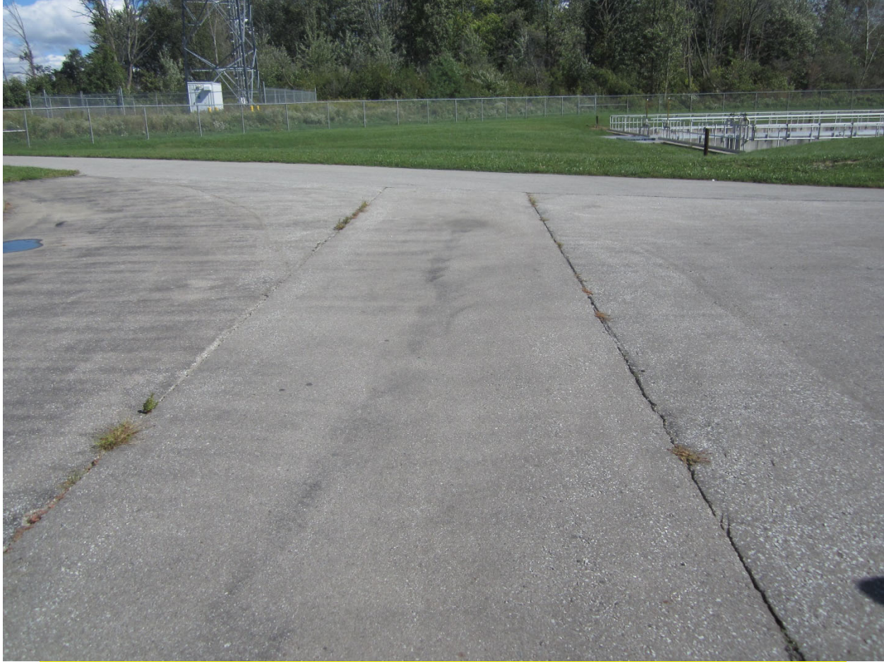
PICTURE OF AREA WHERE NEW BIOFILTER AND HUMIDIFIER WILL BE INSTALLED
