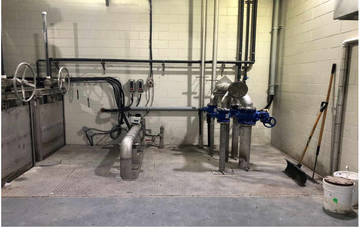
PICTURE OF THE INFLUENT CHANNEL AFTER ASR MANIFOLD INSTALLED
