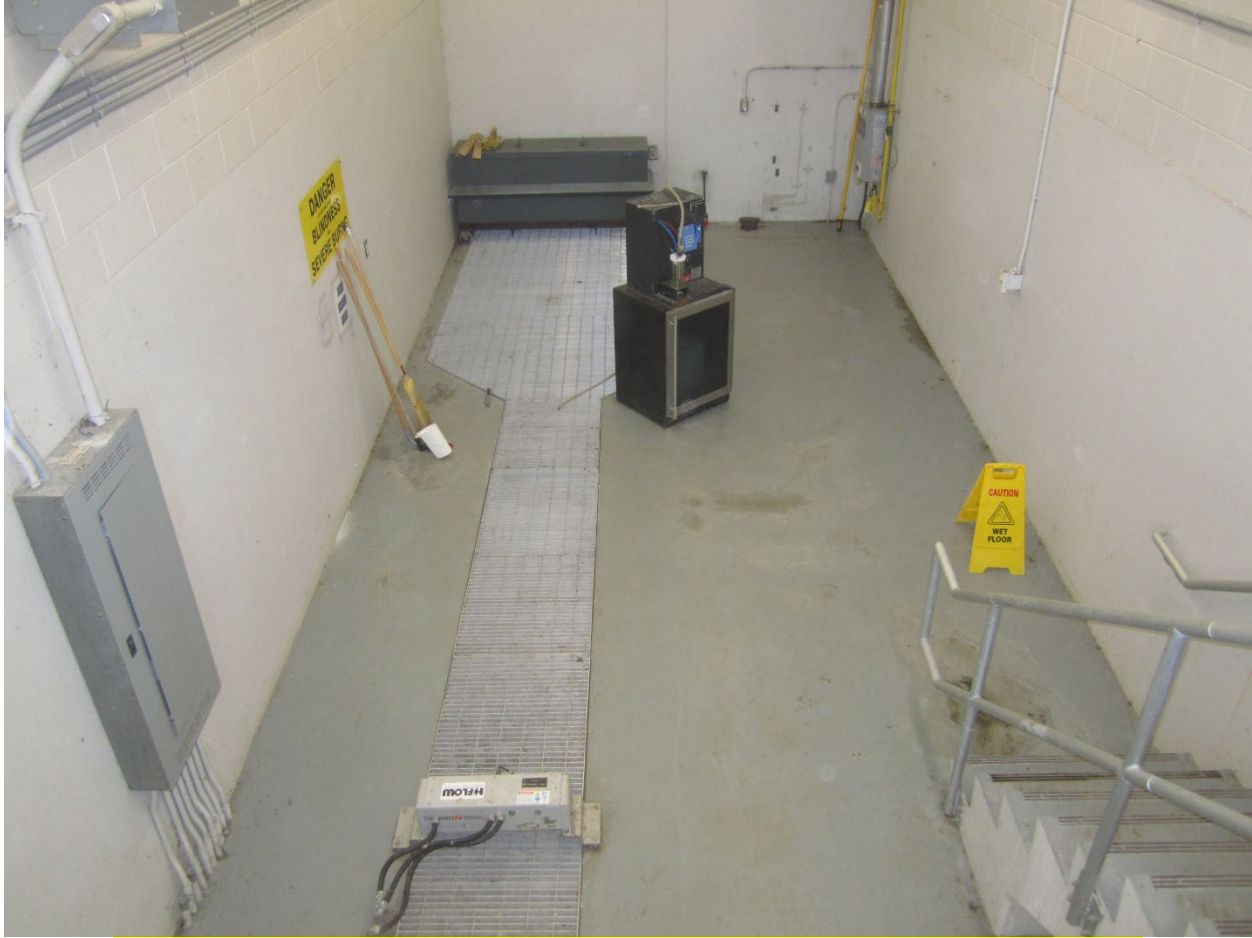
PICTURE OF EFFLUENT CHANNEL BEFORE INSTALLATION OF REUSE SKID
