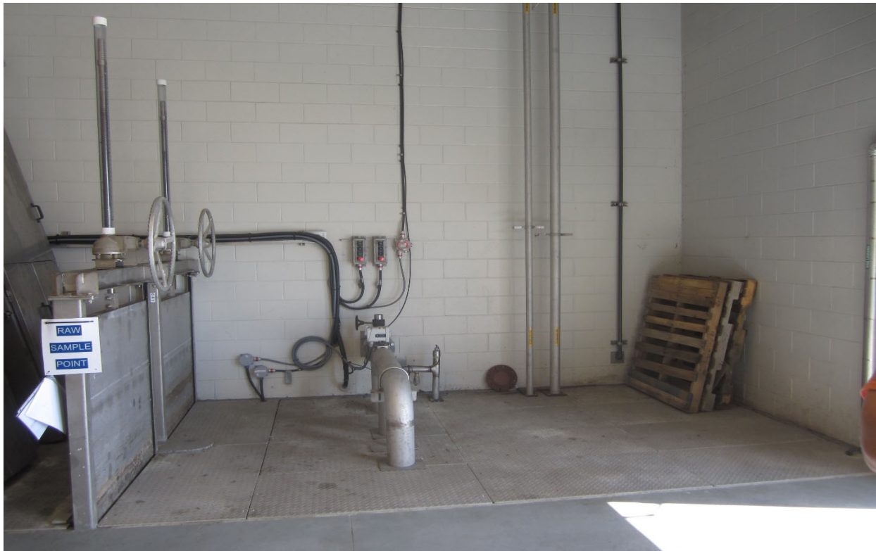
PICTURE OF THE INFLUENT CHANNEL BEFORE INSTALLATION OF THE ASR MANIFOLD
